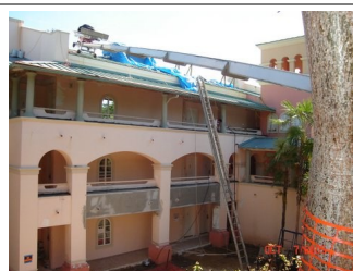
Front roof staging area
