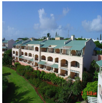
Rear view of roof area
