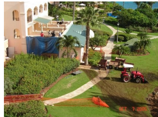
Construction in progress
