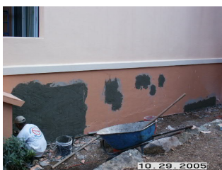
Concrete wall repair
